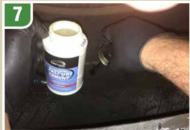
7 Apply PRC Chemical Vulcanizing Cement and allow to dry.
