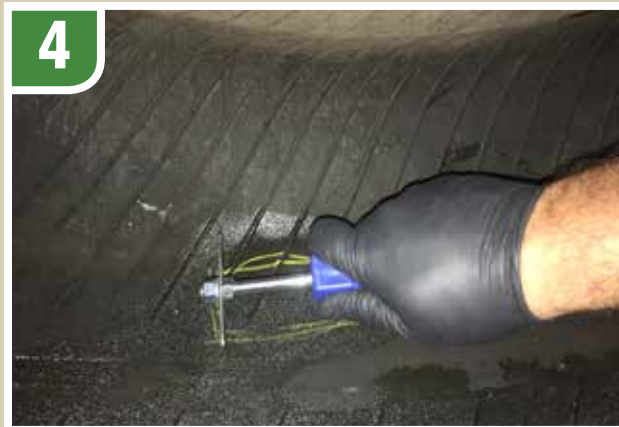
4 Scrape area clean.
