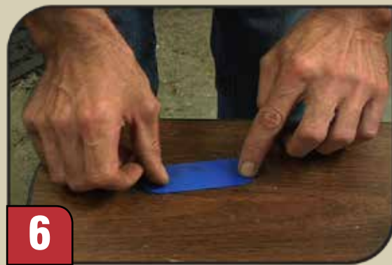
Gently twist Primer Gum and place on 6" packaging tape.
