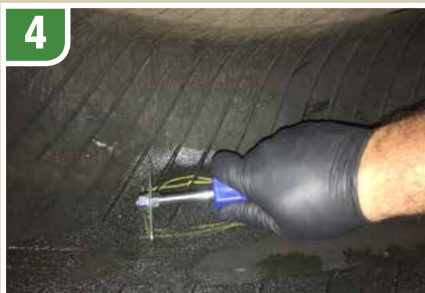
4 Scrape area clean.
